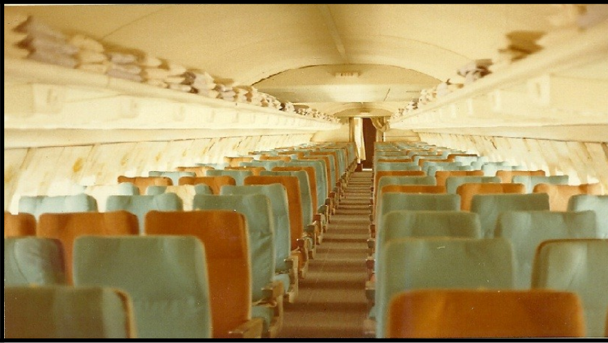
The Cabin on an all Economy B707. The overhead racks pretty much from where the photo was taken, aft, were badly buckled and bowed.
